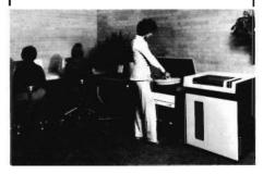
THE DESIGN FEATURES of the system can suit any office location. Pictured above is a standard configuration consisting of 32K of memory, three 2236D terminals, one floppy disk and ten megabytes of disk storage with a 240 line-perminute printer.
